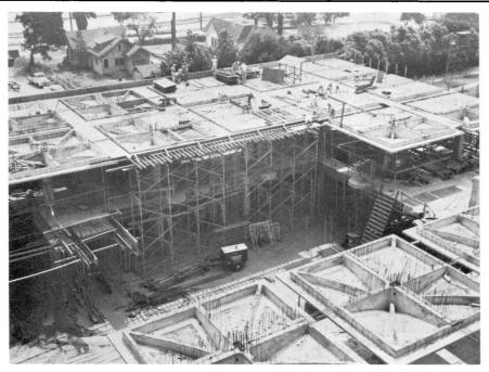
PROGRESS PHOTO—In this unique photo, taken from the TOP of the huge crane at the construction site, you can see the massive concrete umbrellas beginning to form the roof of Ambassador's new Dining Hall.
